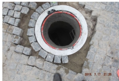
Levelling with floor
