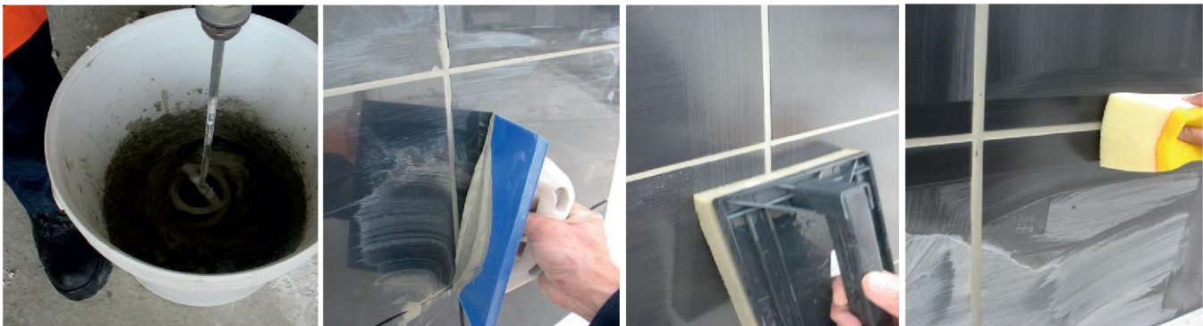
Mixing of ADHERE Cor 05
