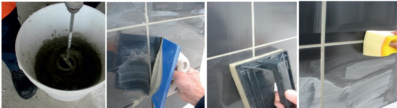
Mixing of ADHERE Cor 312
